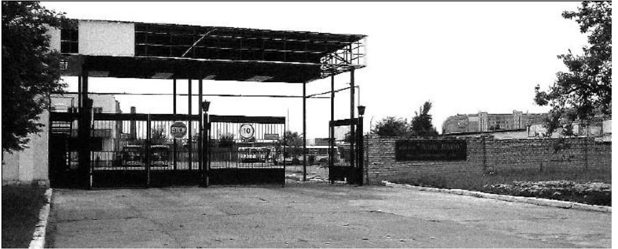
“Alan-techno” bus station
